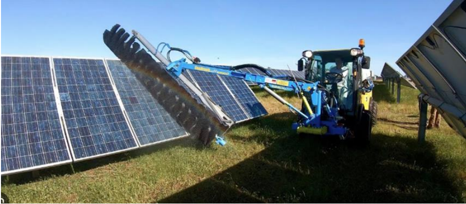
Insert 44: Cleaning of Solar Arrays
